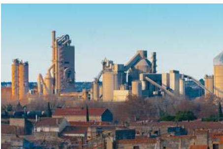
Cement Industry Rotary Kiln & Vertical Shaft Kiln, Clinker
