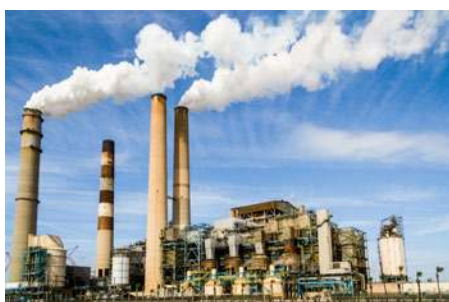
Paper And Pulp Industry Digester, black liquor storage, recovery boiler.
