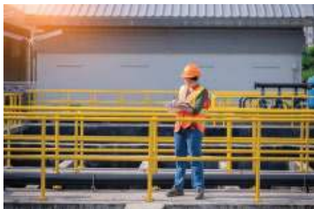
Wastewater Treatment Plants Sludge storage and anaerobic digestion
